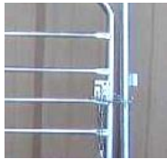
Latch options for gates: vertical, chain and spring loaded latches.
